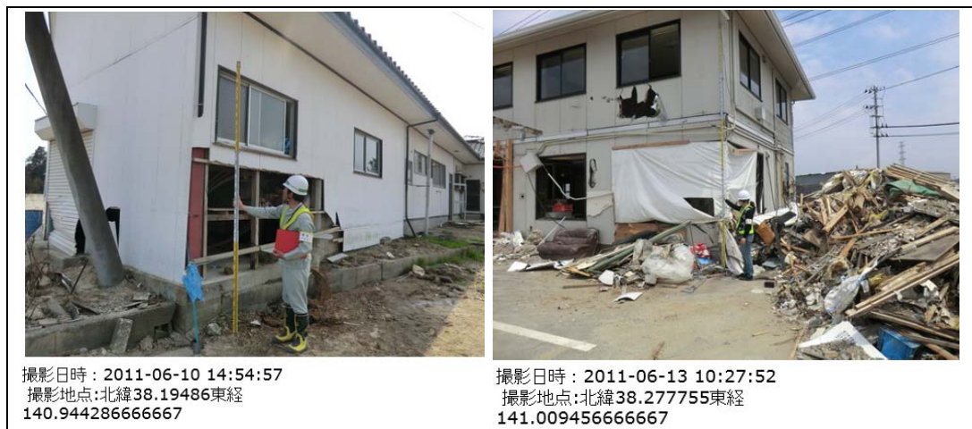
Figure 6.7. Measurement of height information as given in the dataset water marks. Photography available on http://fukkou.csis.u-tokyo.ac.jp/ , Copyright © 2012, Reconstruction assistance research archive secretariat.
