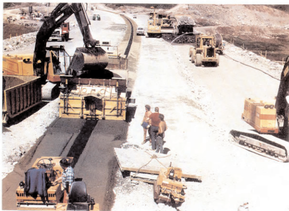
Fig. 2.1 Asphaltic concrete core construction for Riskallvatn Dam
