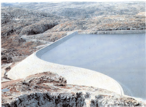
Fig. 5.1 Photo of Storvatn Dam showing the unusual alignment
