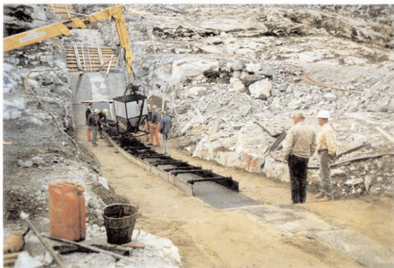
Fig. 4.6 Hand placement of asphaltic concrete
