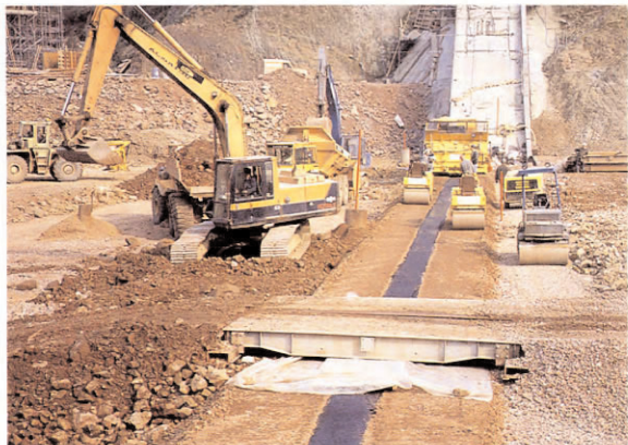
Fig. 4.8 Light steel bridge across the core
