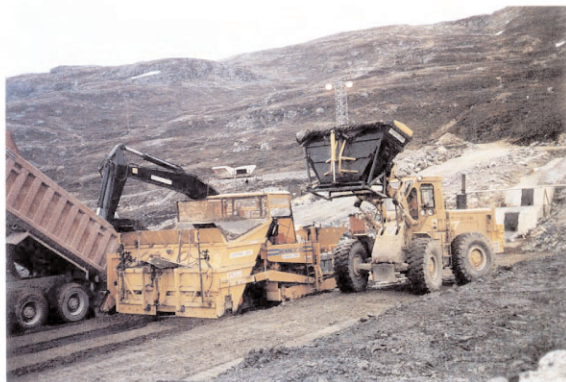
Fig. 4.5 Loading of asfaltic concrete and filter material into paver
