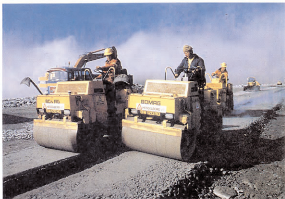
Fig. 4.4 Simultaneous compaction of core and filters
