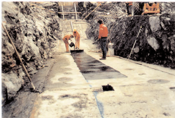
Fig. 4.7 Placement of asphalt mastic on the foundation sill
