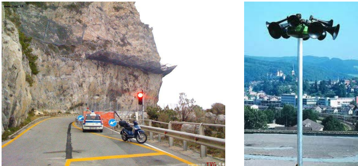
Figure 36: Traffic lights can stop car traffic during high hazard level (Capo di Noli, SV, Italy) while sirens can transmit evacuation signals (Canton Ticino, Switzerland).
